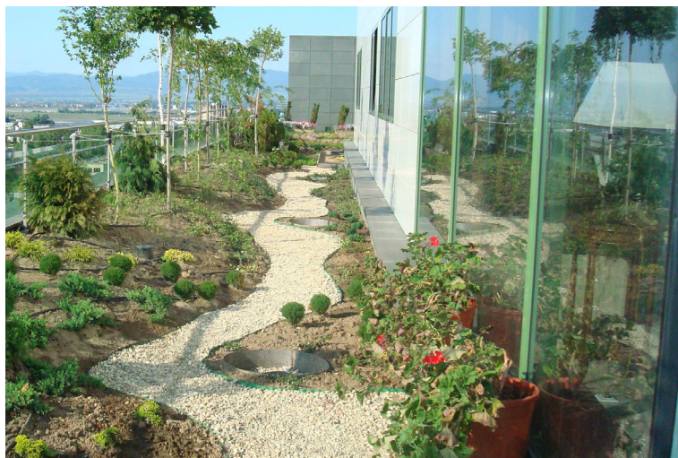
Application of EshaGum Antiroot anti-root membrane, Sofia, Bulgaria.
