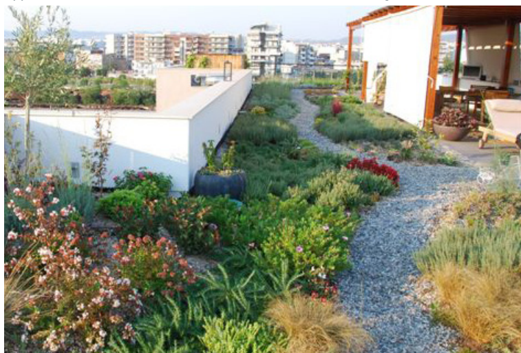
Application of EshaGum Antiroot anti-root membrane on a roof in Thessaloniki.
